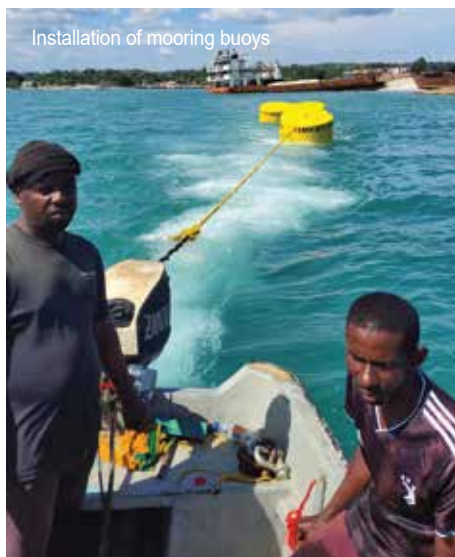
Pull test mooring systems
