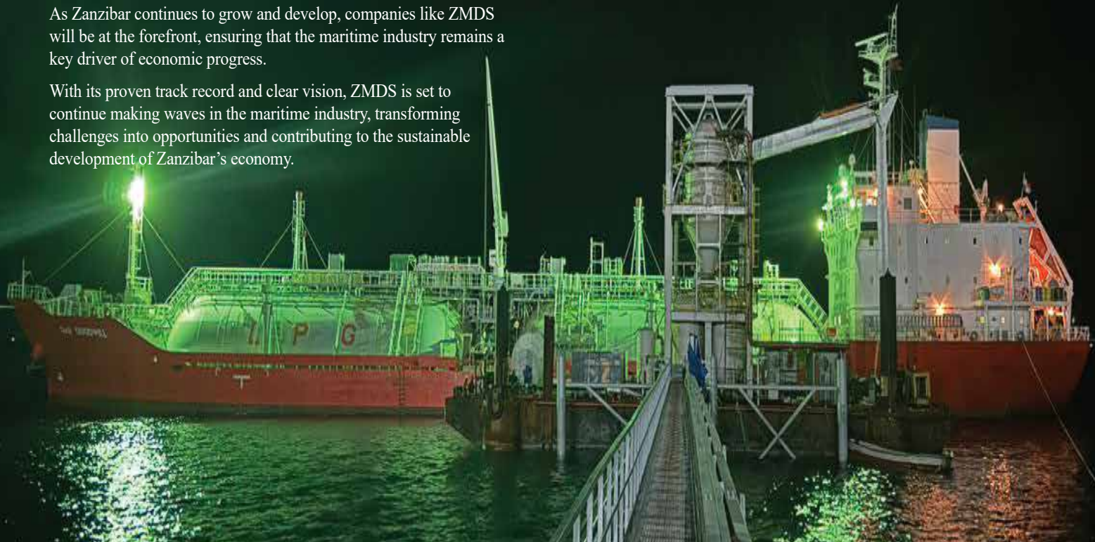
installation of Barge platform on jetty
